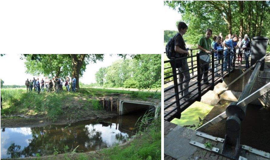
Figure 17 Trade-offs and synergies with the surrounding land use: a culvert (left) controls the discharge in the restored channel and a weir (right) is still in operation to regulate water levels for the surrounding agriculture
