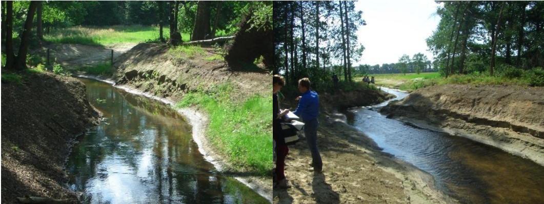
Figure 16 Excavating the former channel
