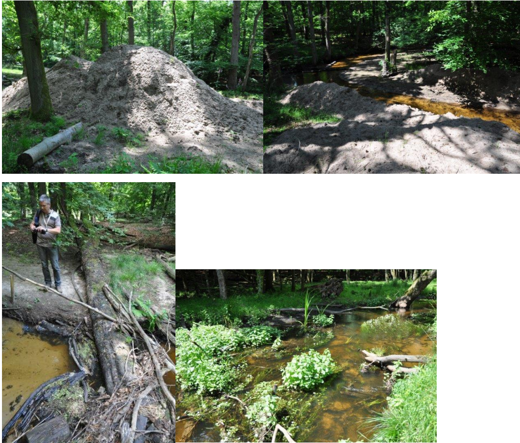
Figure 7 Sand supplementation (top); wood addition (bottom)
